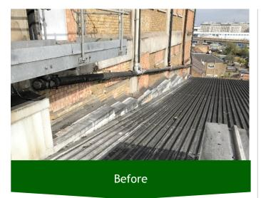
The existing up stand was covered with mineral felt, the felt was failing throughout and coming away from the curb, it was extremely dirty and covered with traffic film and sticky residue fall out from the refinery.
