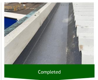
Once all cleaning and preparations has been completed as per the manufacture's guidelines, operative fully encapsulated the full length of gutters with the Giromax Girolsil® RC-G coating to complete the treatment,
