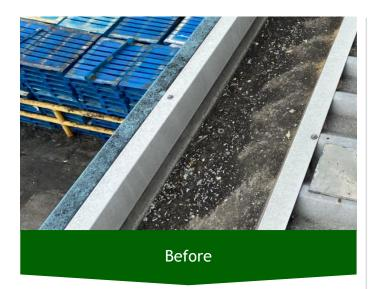
The existing gutter liners were heavily soiled and varied in level of corrosion, it was evident that the gutter joints had leak throughout causing water staining on the cladding below.
