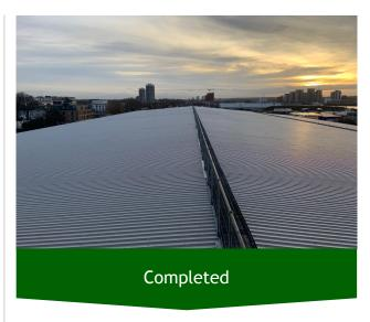
Once all cleaning works had been completed, all lap joints were sealed using Giromax Girosil® SE and then then all areas that had cut edge corrosion treatments where primed including encapsulating all fixings.
