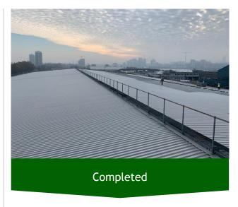
All roof voids left from their removal where over sheeted with matching steel roof sheets both externally and internally prior to the roof coating system being applied to leave a seamless consistent finish.
