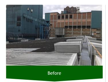
The smoke units had been causing water ingress issues throughout the warehouse and packing hall directly below.
