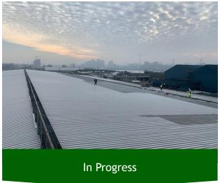
The roof surfaces had to be thoroughly cleaned at high pressure to remove the build up of the thick dirt and grime that had accumulated on the roof over many years.
