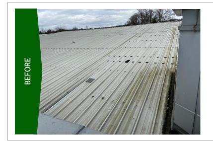
The existing roof sheets were dirty and there was evidence of historical patch repairs throughout, cut edge corrosion was present on the sheets which had caused the original factory applied coatings to start peeling back exposing the steel substrate.
