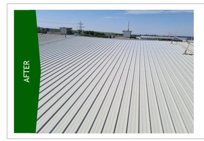
Once all the relevant preparation works had been completed to the roof area which included all roof sheets, flashings and capping sections. The Liquasil MetalSeal 20 roof coating system was applied via airless spray as per manufacturers specification.
